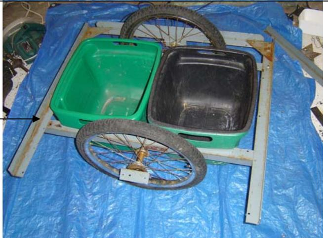
13. Place the right edge of the bed frame (cut off at the start) into position, then drill and bolt it to the bed frame and the right hand 100mm wheel support. Again ensure the wheel and wheel support is as straight as possible and the trailer is square. Use four 6mm x 20mm bolts.
