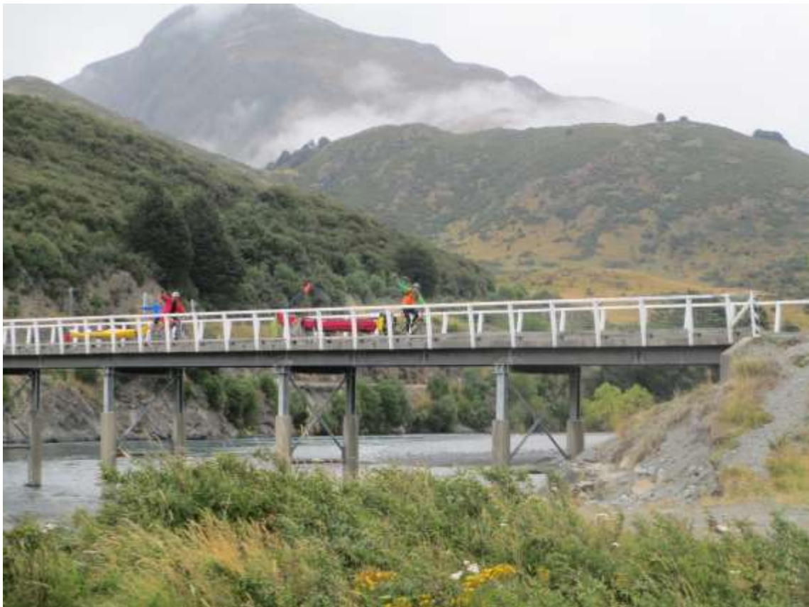
Crossing Mt White Bridge
