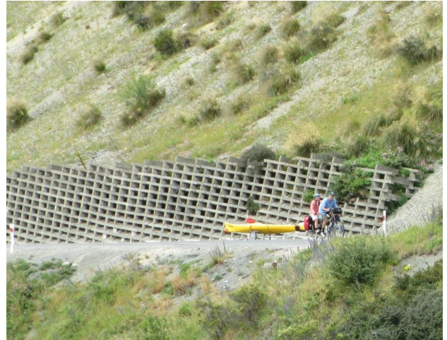
Olly & Ting nearing the top of Porter's Pass
