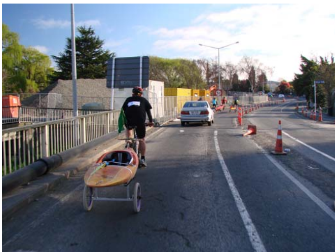
Travelling on earthquake damaged roads
